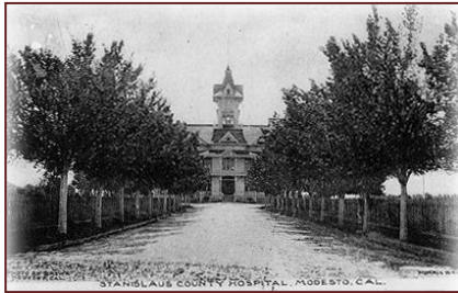
The Alms House was the original home of the Health Services Agency.
